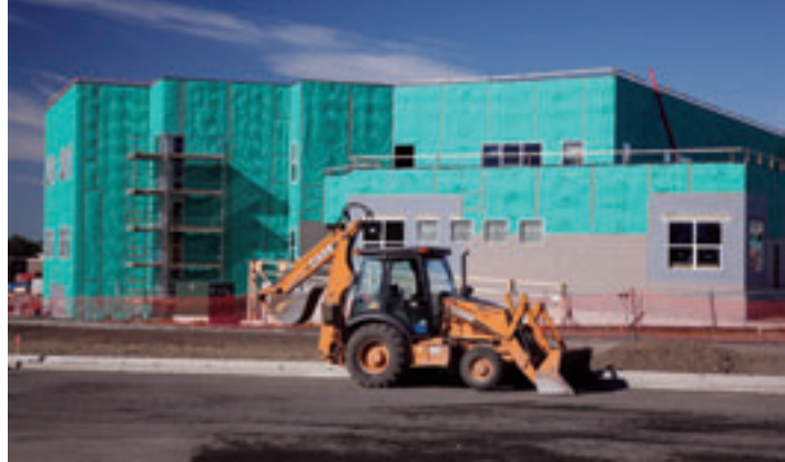
Clark Middle School, Anchorage
