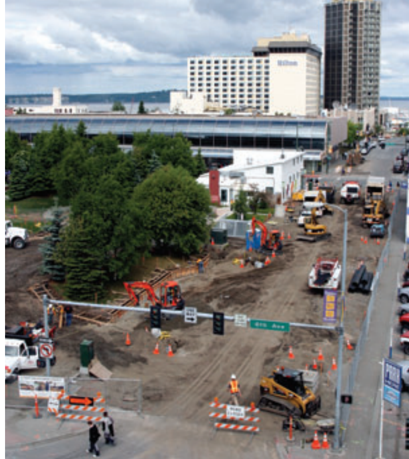
E Street Improvements, Anchorage
